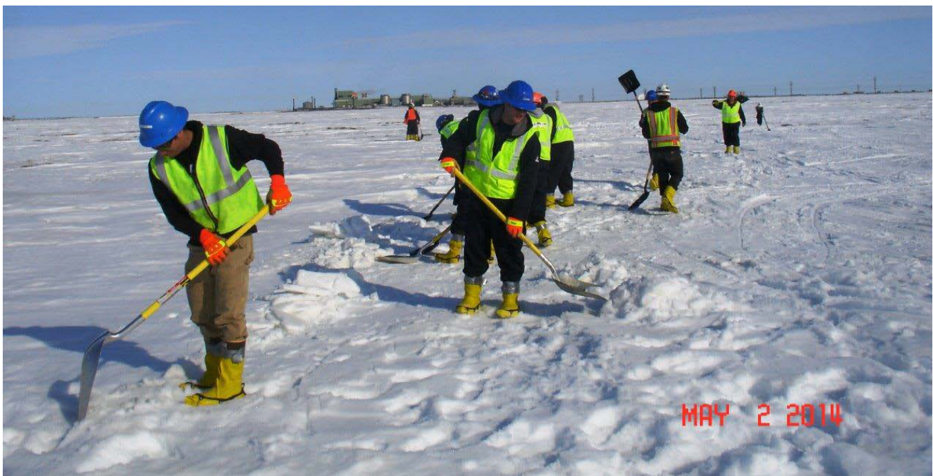
Cleanup workers searching the area for additional oil-contaminated snow. May 2, 2014 (photo: Ebel, ADEC)
