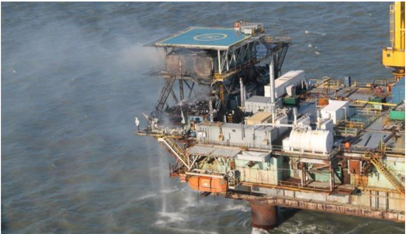
Firefighters applying cooling water on the rig to control flare ups, October 2, 2014. (Photo/Nikiski Fire Department)
