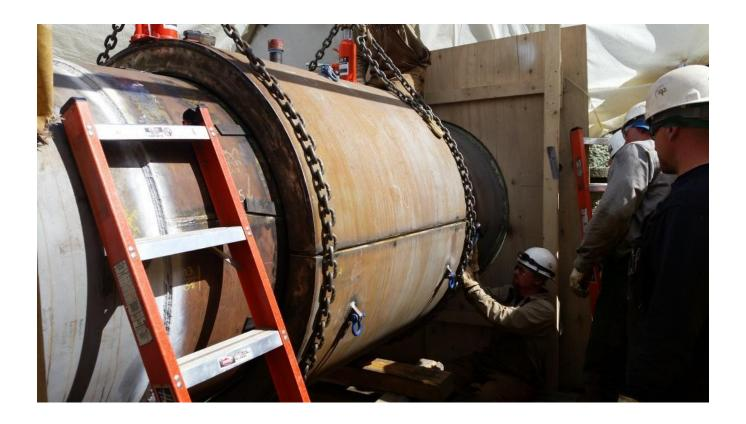
60-inch repair sleeve fit-up complete over line. (Photo: Alyeska Pipeline Service Company)
