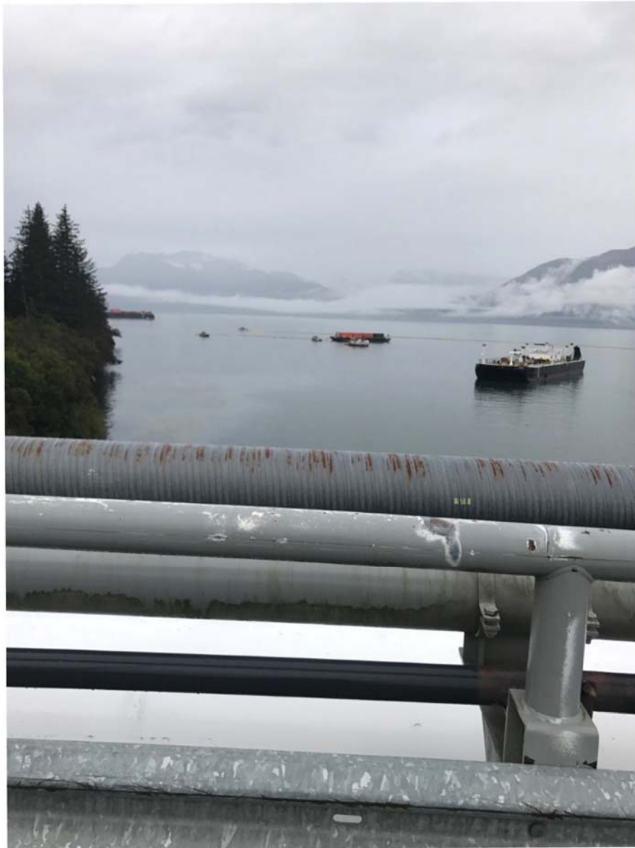
Photograph from Berth 5 facing west, taken by ADEC Responder
